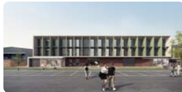
Centre for Green Technology building currently under construction
