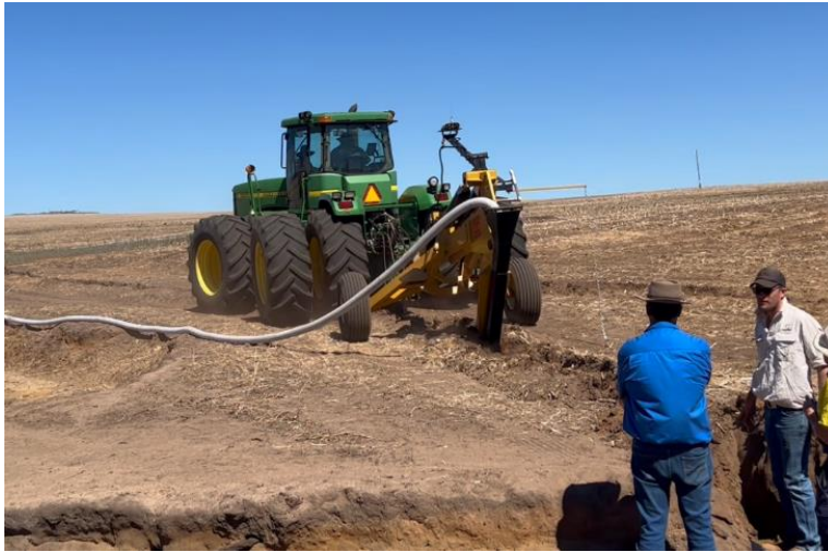
Figure 11. Photograph of the “Soil Max” tile plough installing pipe behind a DGPS-guided tractor during a demonstration field day (note – photo is not at the Webb property, but from a field day).
