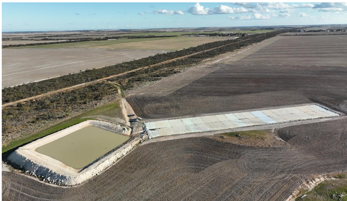
Figure 7. Drone image of WSD Lester site tarped catchment system, May 2023
