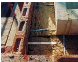
Super-insulation with wall tie
