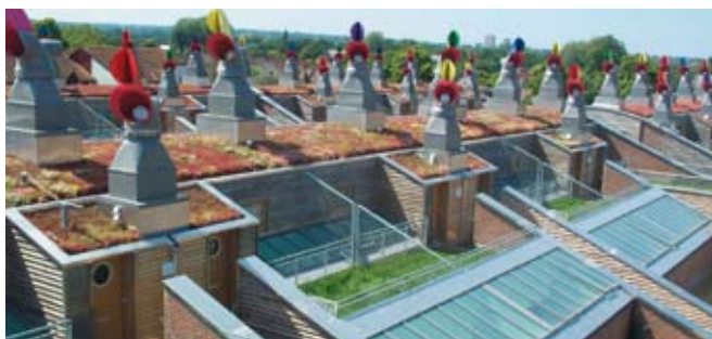
sedum roof and grass turfed sky gardens
