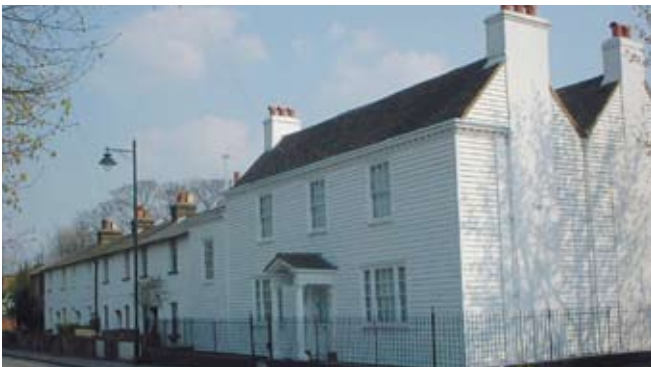
Local historic weatherboarding
