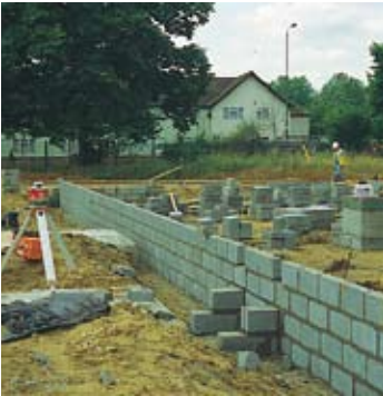
Concrete blockwork at BedZED
