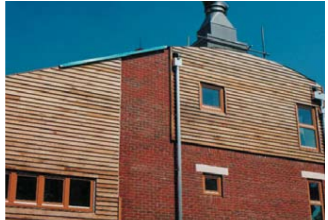
Brick and weatherboarding – west elevation
