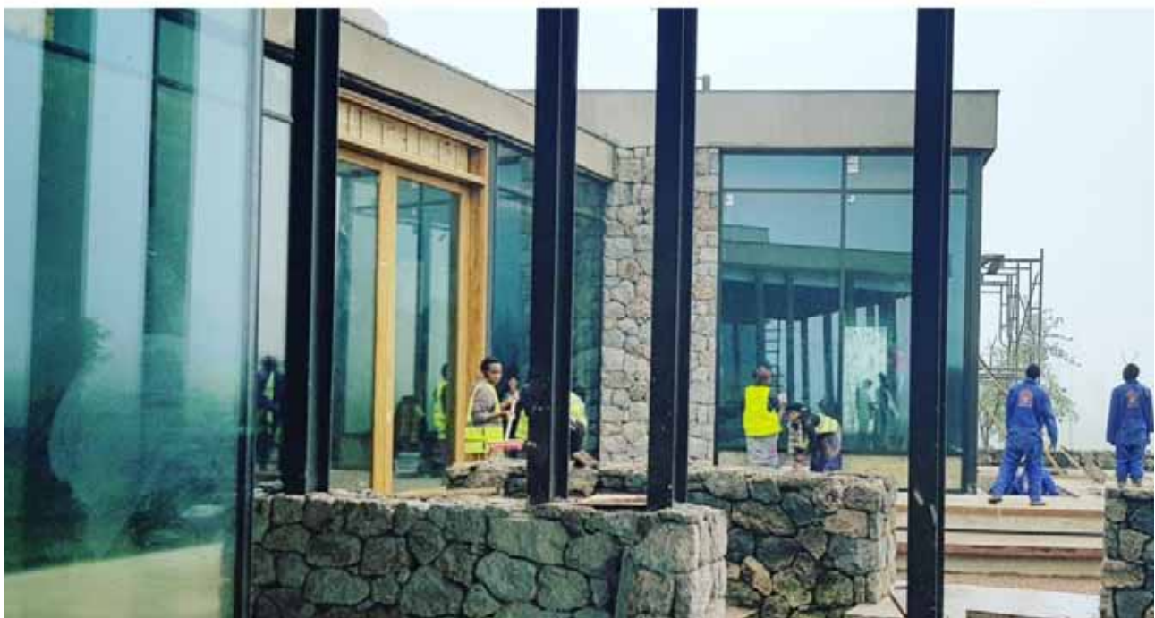
Main Lodge double glazing units during installation
