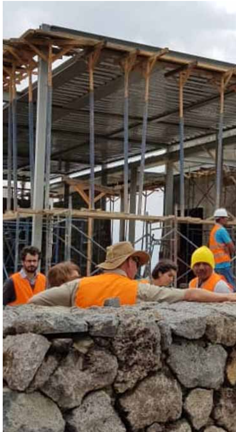
Core building shell construction; steel frame and concrete slab roof
