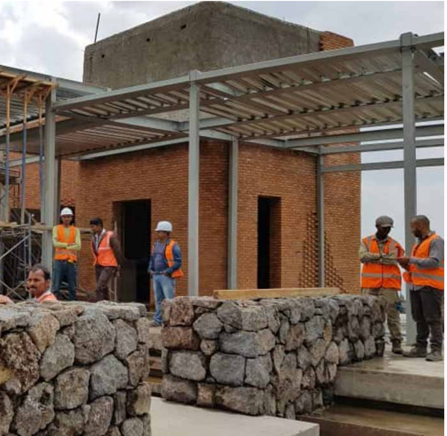
with permanent shuttering
