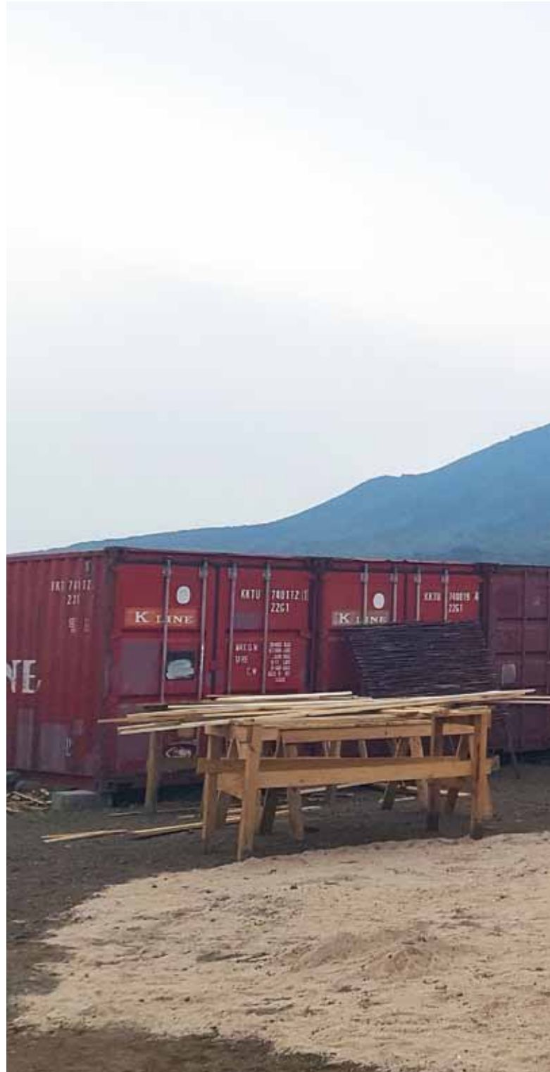
The Site Protection Plan clearly set out material storage and construction
