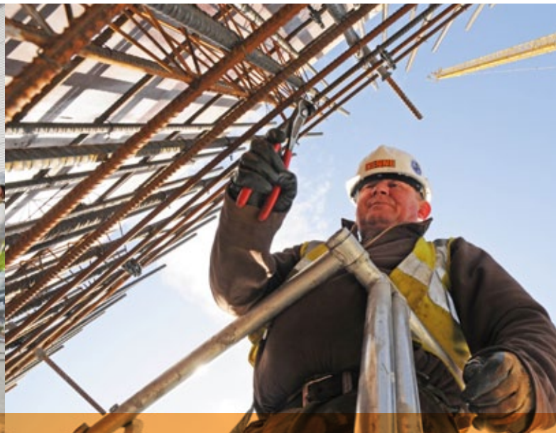
Pouring the green concrete frame
