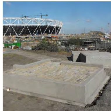
Reclaimed yellow stock bricks used to create seating areas on the Greenway
