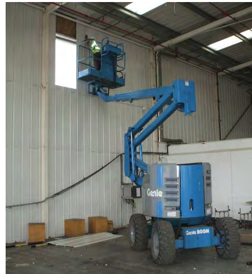
Reclamation of a steel portal frame building on the Olympic Park
