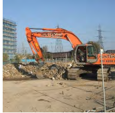
A combination of machinery and manual work was employed in the demolition and reclamation of bricks
