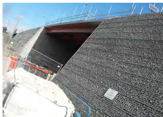
Gabion baskets installed at the LO3 Bridge
