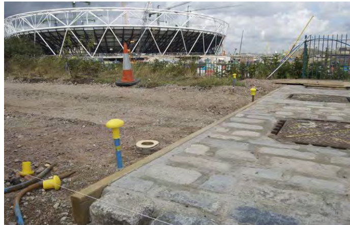
Granite setts being installed on the Greenway
