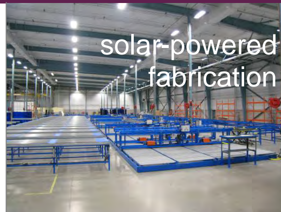
Solar-Powered Panelized Frame Factory on Site
