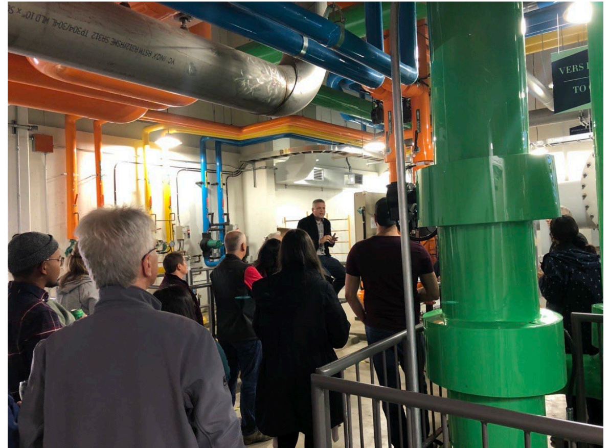
Tour of the ZCU Central Plant © Zibi
