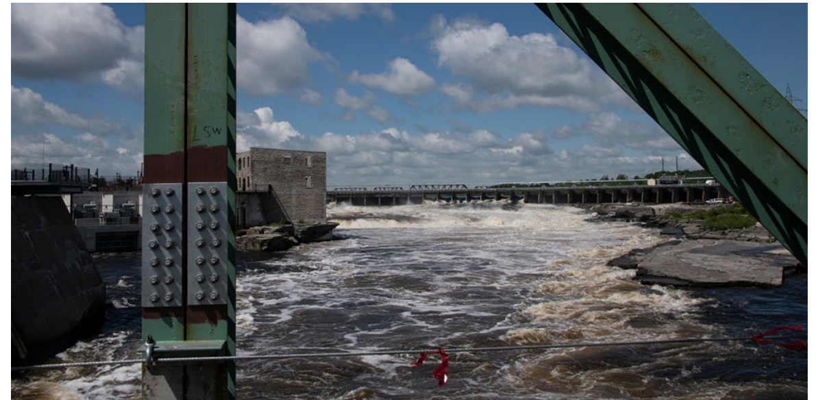
Chaudière Bridge © Zibi
