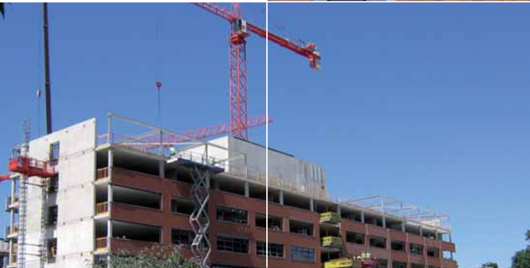
Kingspan - Mid Kent College, pre-fabricated light steel framed panels
