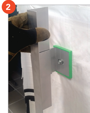
Set depth of installation of rail into bracket based on wall cavity depth
