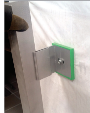
Set depth of installation of rail into bracket based on wall cavity depth
