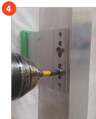
Single Bracket "sliding point" install – fasteners in 2 slots
