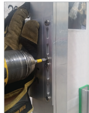
Double Bracket "fixed point" install – fasteners in 4 holes
