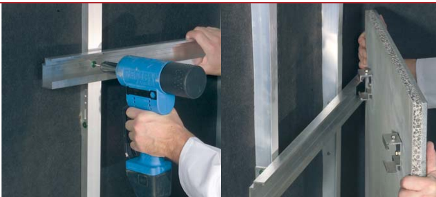
The natural stone composite panels are fastened into the special profiles of the aluminium substructure.
