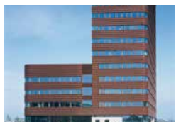
PSG Copper Tower Nordre, Copenhagen, DK Arkitema K/S, Copenhagen NCC Construction A/S, Hellerup TECU® Classic
