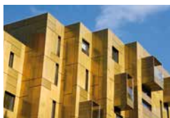
Walpole house, London, UK Make Architects, London CGL Systems Ltd, London TECU® Brass
