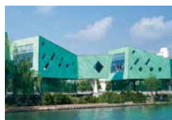
Yefei's Creative Street, Shanghai, SG Will Alsop Architects, London, GB; U/Jiang Architects & Engineers, Shanghai Hanchang Industrial Development Co., Shanghai TECU® Patina, TECU® Oxid, TECU® Bronze
