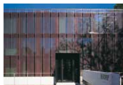
Office building of the International Ice Hockey Federation, Zurich, CH Tilla Theus und Partner AG, Zurich Scherrer Söhne AG, Zurich TECU® Classic_flatmesh
