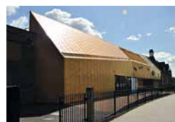
Pegasus Academy's Whitehorse Manor School, London, UK Architect Hayhurst and Co., London, UK Richardson Roofing, Staines upon Thames, UK TECU® Gold
