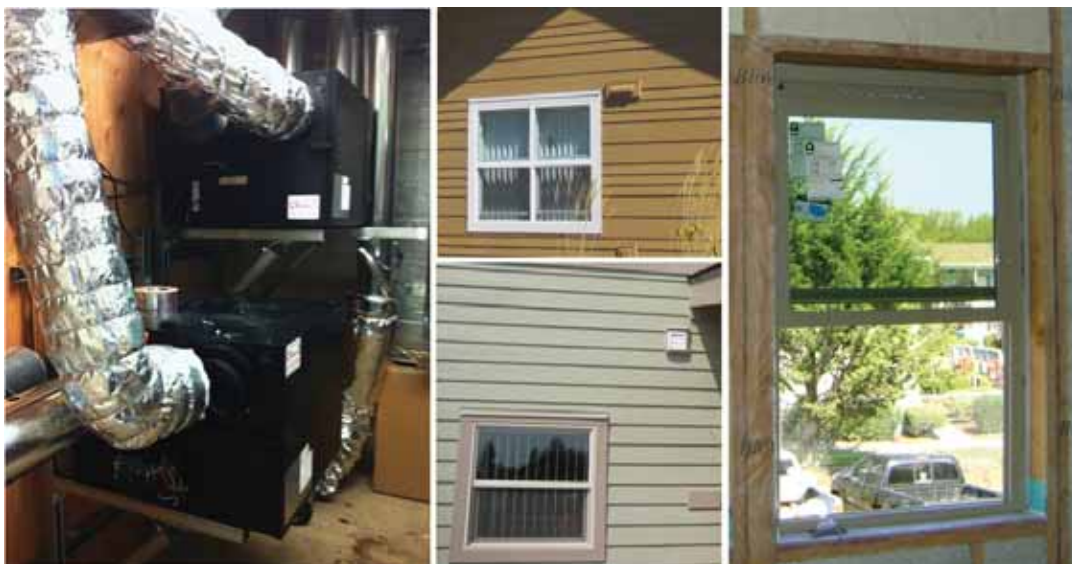
Figure 6: ERV at PH (left), examples of passive air inlets (center), trickle vent at window head at EA (left: Kwok 2014, center and right: Author 2013).
