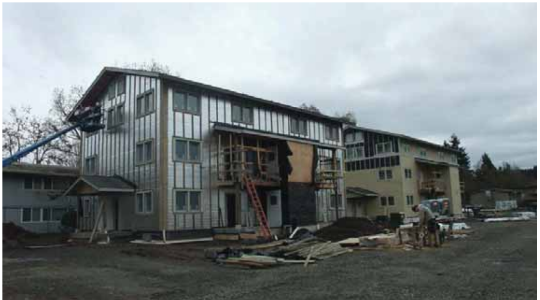
Figure 2: Continuous insulation over WRB on PH (left), siding directly over WRB on EA (right).
