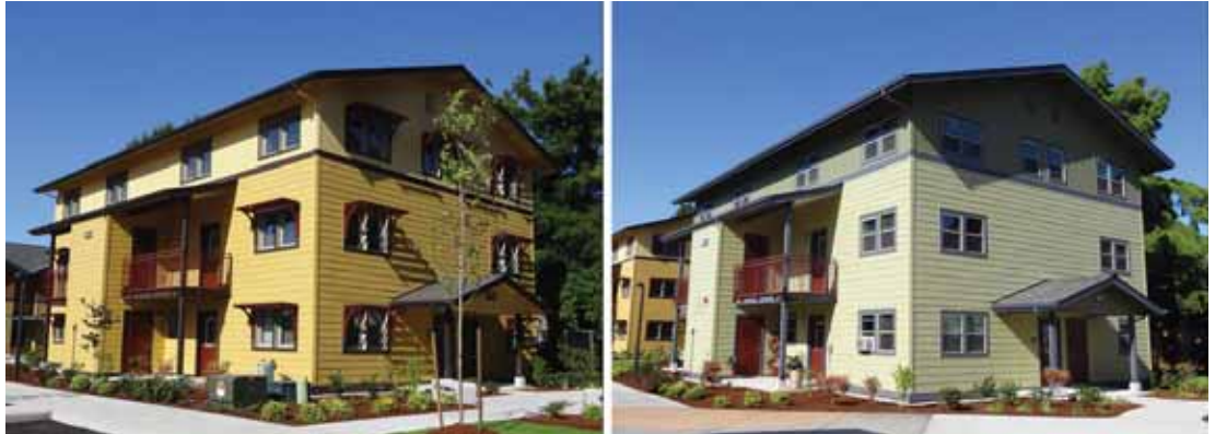
Figure 1: Passive House case study building (left), Earth Advantage case study building (right).
