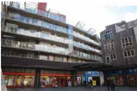
Figure 8: Gallery Access at the commercial courtyard
