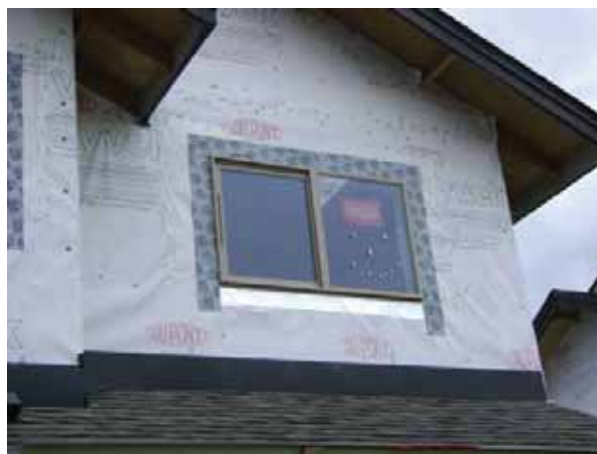
Figure 5: Air barrier house wrap with taped seams at PHIF.
