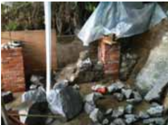
Figures 6, 7 and 8: The natural stone wall here is not a dry wall, but rather bound by mortar.
