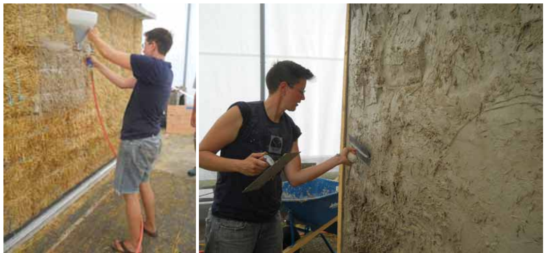
Figure 3: Spraying clay slip (drywall texture gun and air compressor) and two-hand trowel plaster method.
