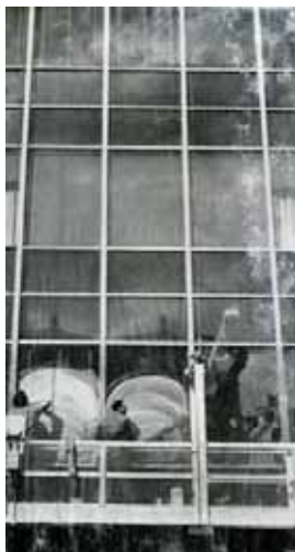
Figure 6: Lever House window washers. Source: Architectural Forum, June 1952
