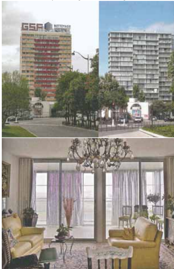
Figure 7-8: Frédéric Druot, Anne Lacaton, and Jean Philippe Vassal, Transformation of Tour Bois-le-Prêtre, Paris, France, 2006–11 displayed at 'Small Scale, Big Change. New Architecture of Social Engagement' exhibition. New loggias, built as self-supporting structure, are added on three sides of the building. The transformation of the residential tower shows the legitimacy of the thesis architects disclosed in their study PLUS in 2004. Source: (Ciorra, Marini 2012, 26-27)
