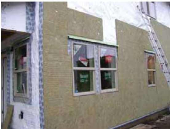
Figure 3: Continuous insulation over WRB on PHIF.
