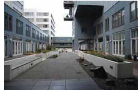
Figure 6: The West courtyard at De Zilvervloot with social housing on either side.
