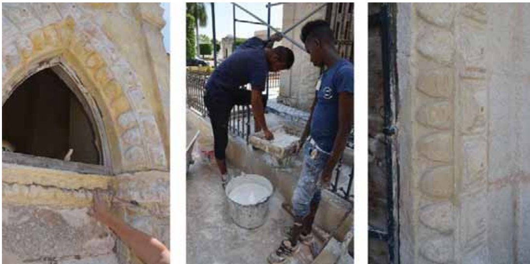
Figure 4: Escuela Taller students at work on a project in the Colón Cemetery. The trade skills these disadvantaged youth learn on projects such as these are valuable in the preservation profession. Source of image: (Author, 2014).
