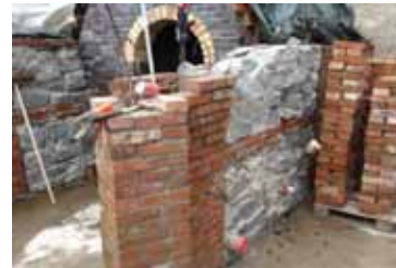
Figures 6, 7 and 8: The natural stone wall here is not a dry wall, but rather bound by mortar.
