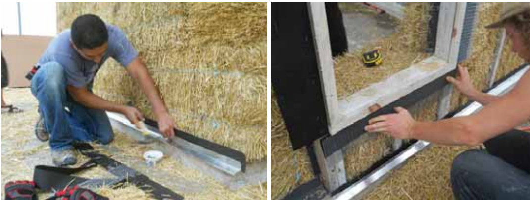
Figure 2: Application of air-fins, flashing, and metal lath at critical transitory locations along the wall plane.
