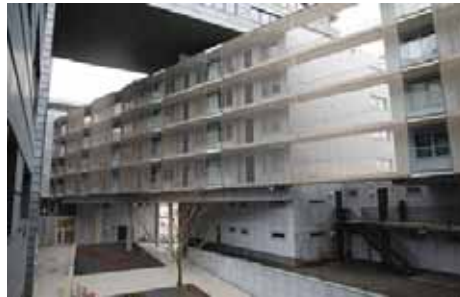
Figure 9: Access galleries at La Grande Cour's East courtyard
