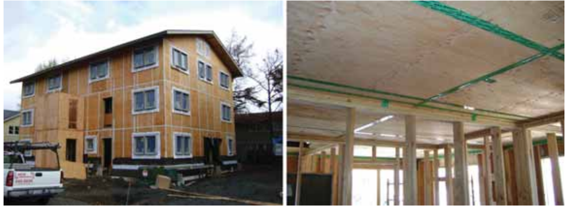
Figure 4: Taped plywood seams throughout PH.
