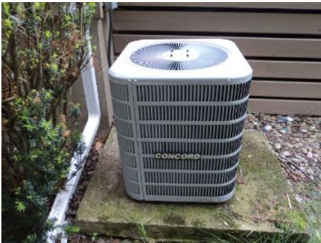
Concord AC Unit - Model# 4AC13L30P / Serial# 1913A20538
