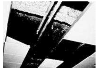
Sprayed asbestos on steel beam
