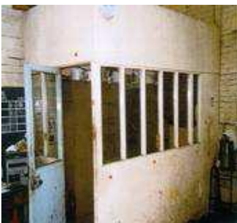
An office made from Asbestos Insulating Board
