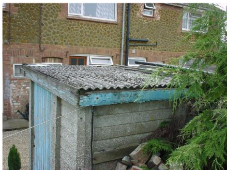
Asbestos Cement roof sheets House clad with asbestos cement Cold water storage tank
