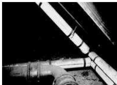
Asbestos pipe lagging in a loft
