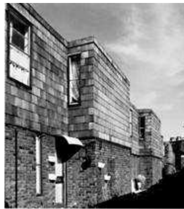
Asbestos cement tiles
