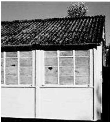
Asbestos cement roof
