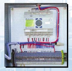
**System PLC** is designed to allow flexibility in C&C applications. It monitors dust accumulation and operates the conveyor only as needed to save energy.
