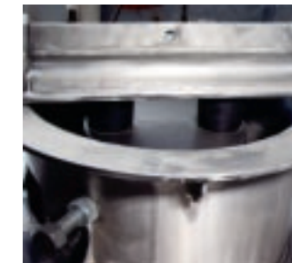
Top-Mounted Isolation Springs
