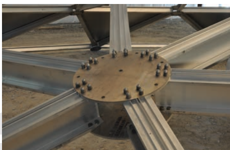
Node detail utilizes proprietary extrusion design.
