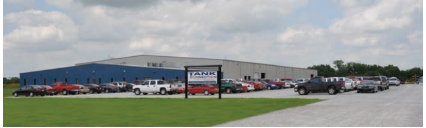
Tank Connection's 85,000 sq. ft., state-of-the-art manufacturing facility was brought on line in early 2009. The facility commands the top position in bolted tank manufacturing worldwide!
