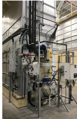
Material handling mill conveyor
