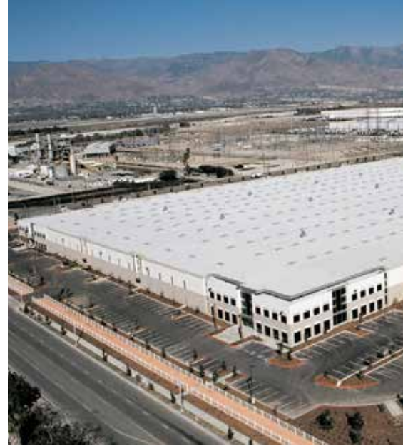
Redlands, CA: Est. 2006 16 acres under roof (684,000 sq. ft.) • 35 acre site
