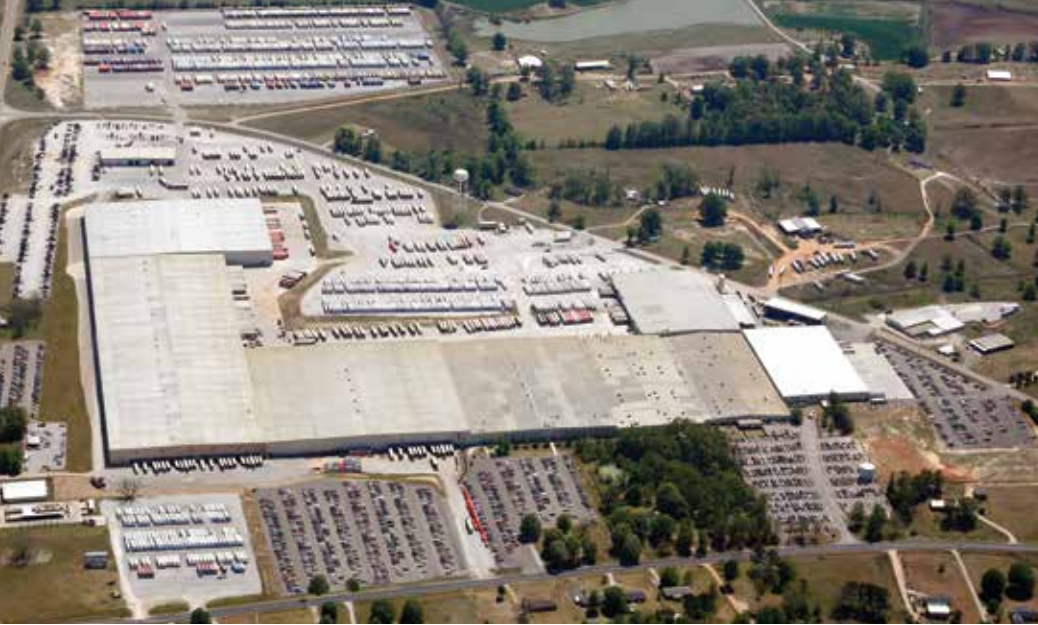
Ecu, MS: Est. 1994 - WORLD'S LARGEST UPHOLSTERY PRODUCING PLANT 46 acres under roof (Nearly 2,000,000 sq. ft.) • 100 acre site
