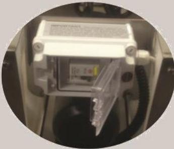
The RCD is located underneath the unit. To reset or test please pull the lid down to open.
