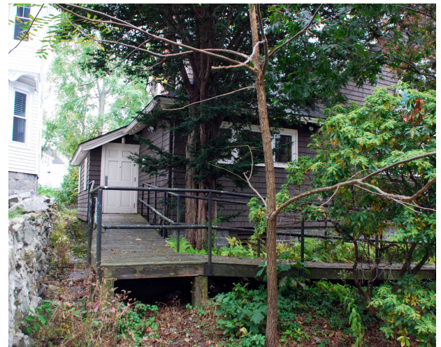
Access ramp is damaged and hidden behind overgrown plantings
