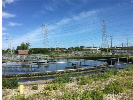
Black & Veatch Corporation prepared a report in connection with the P-removal Feasibility Study for the O'Brien Water Reclamation Plant (NRP WRP). The plant cleans an average of 230 million gallons of wastewater per day (mgd) and has the capacity to treat **450 mgd**. Detailed description of Kaletetch's Engineering's role is summarized in the following:
