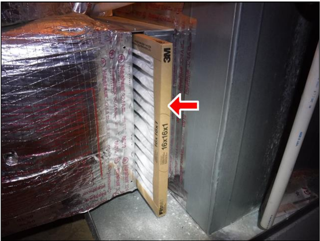
View of air handler filter
