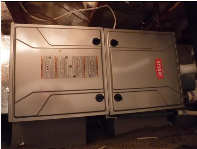
Natural gas furnace, crawlspace, serves first floor
