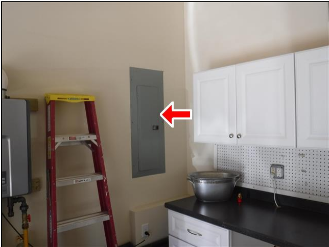
Service panel and main disconnect
