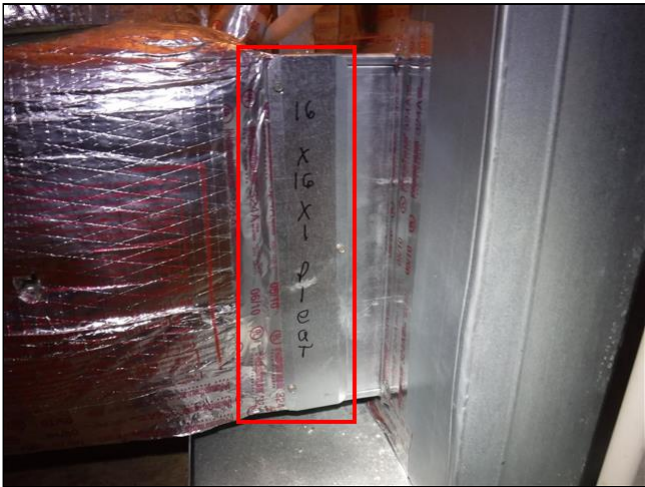
Air handler filter location (serves all of second floor)
