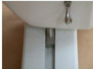
Rear view of Panel with Nut on the Fixing Block, And Hexhead Bolt.
