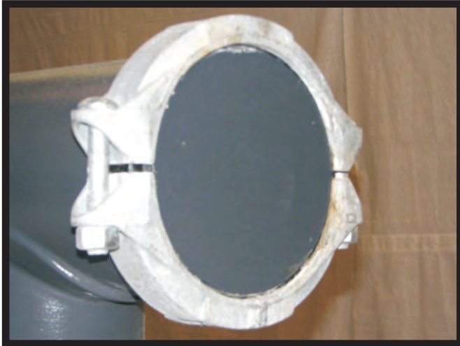
End cap being installed
