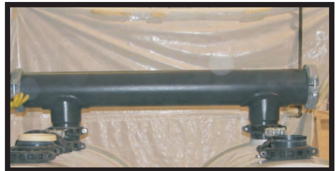
Typical two-branch manifold
