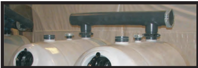
Photo depicts system effluent manifold, positioned in left configuration
