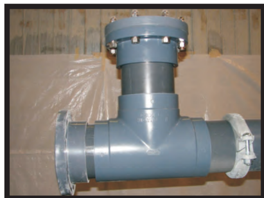
Priority Flow Control Valve into a two-branch manifold
