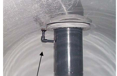
Automatic Air Relief Assembly
