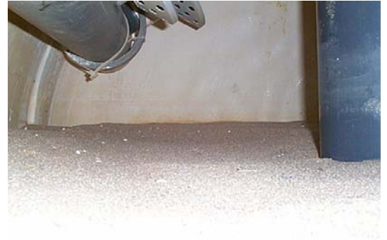
Above: Sandbed should be flat and smooth when sand is installed.
