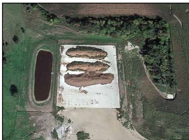
Permanent stockpile facility with concrete pad and runoff pond. (NDDoH)
