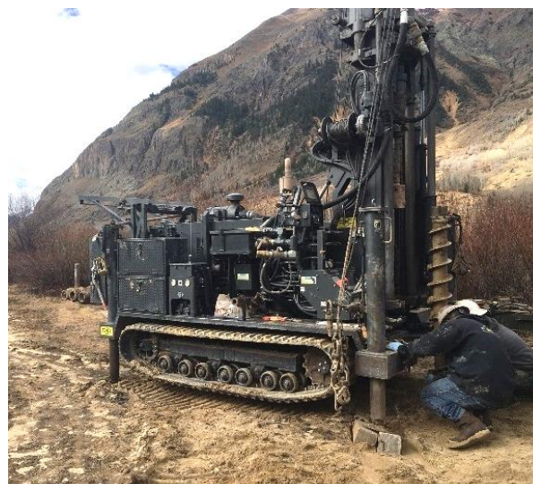
Groundwater well being drilled at the Kittimack Tailings
