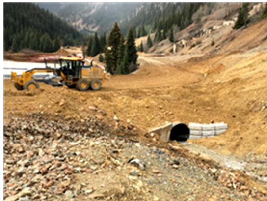
Culvert repair near the IWTP at Gladstone
