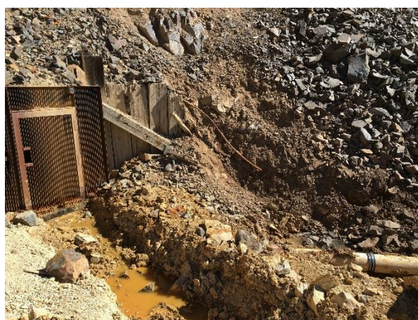
Brooklyn Mine adit with repaired pipeline (lower right)
