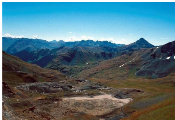
Lake Emma after it collapsed and drained into mine structures below the surface
