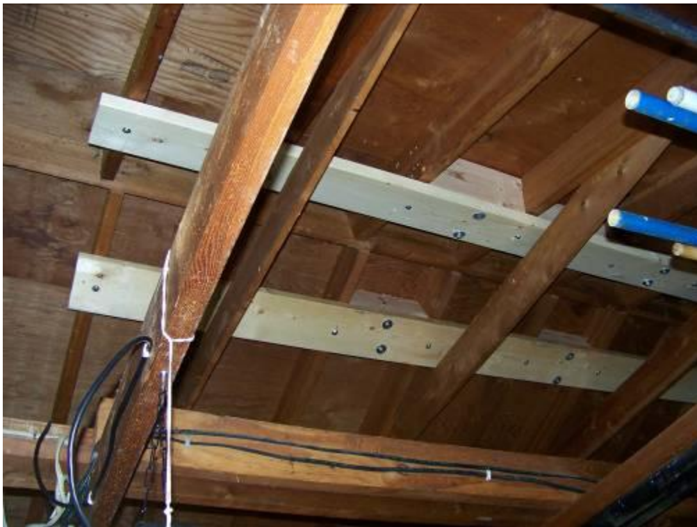
Added roof reinforcement for tower
