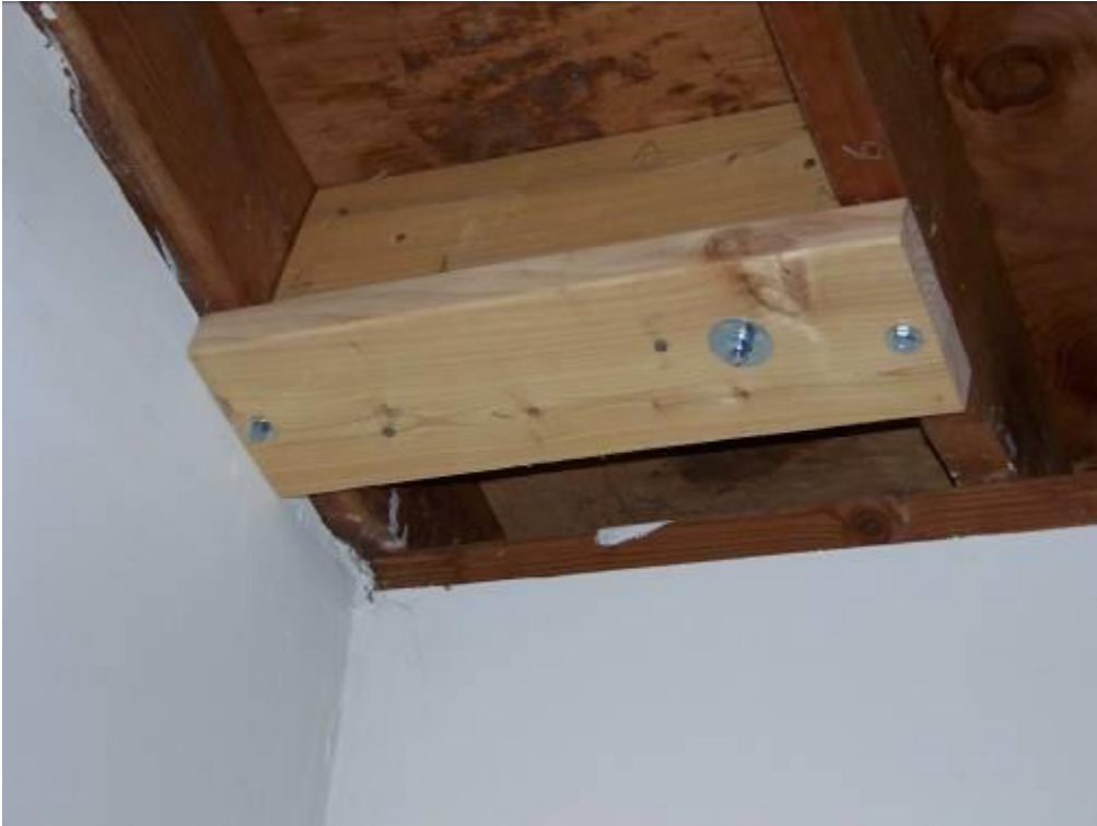
Roof reinforcement for the guy cable attachment points
