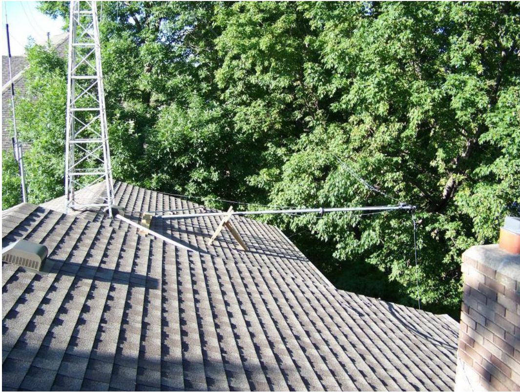
Falling derrick made from two sections of a telescoping TV mast that I have been saving for 35 years.
