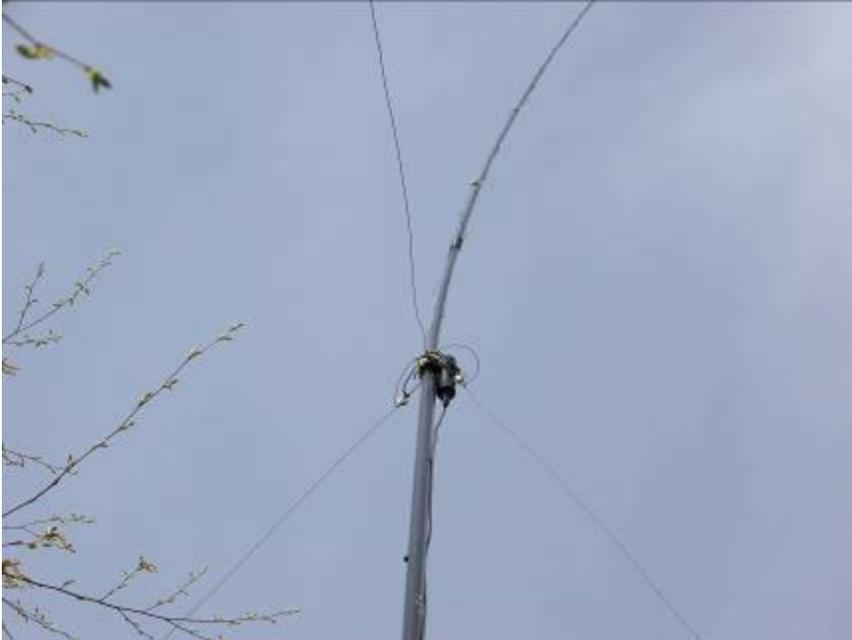
Balun and connection of the radials to the fiberglass pole
