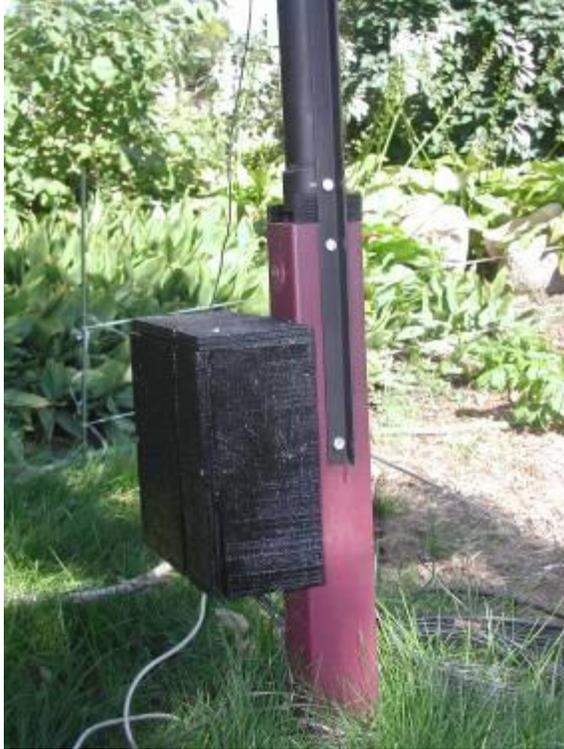
When the structure is horizontal, the bottom bolt is removed. The structure is raised by pivoting on the upper bolt. Once the structure is vertical, the bottom bolt is installed. Installation is a bit tricky because a small motion at the bottom bolt results in a large motion at the top of the structure (45 feet up).
