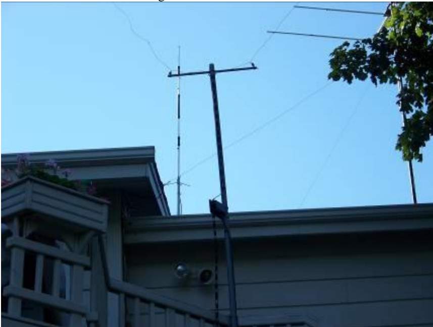
The ten meter band tap with the ladder line going below the deck for earth ground connection.
