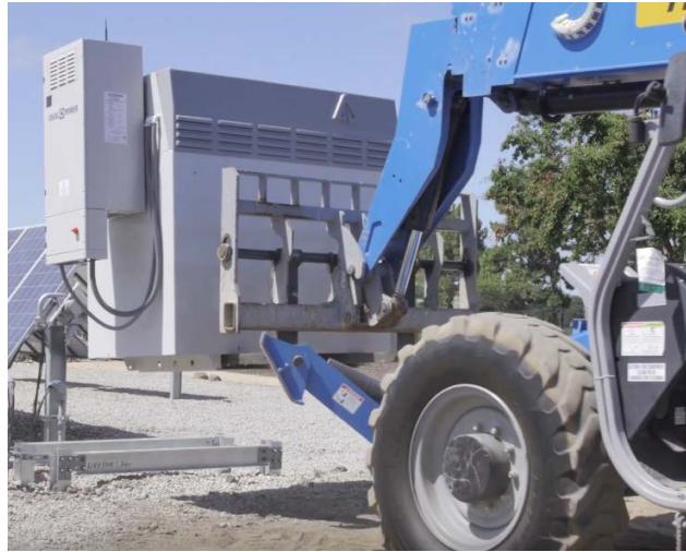
Figure 6 – Example of battery being handled via fork lift pockets.
