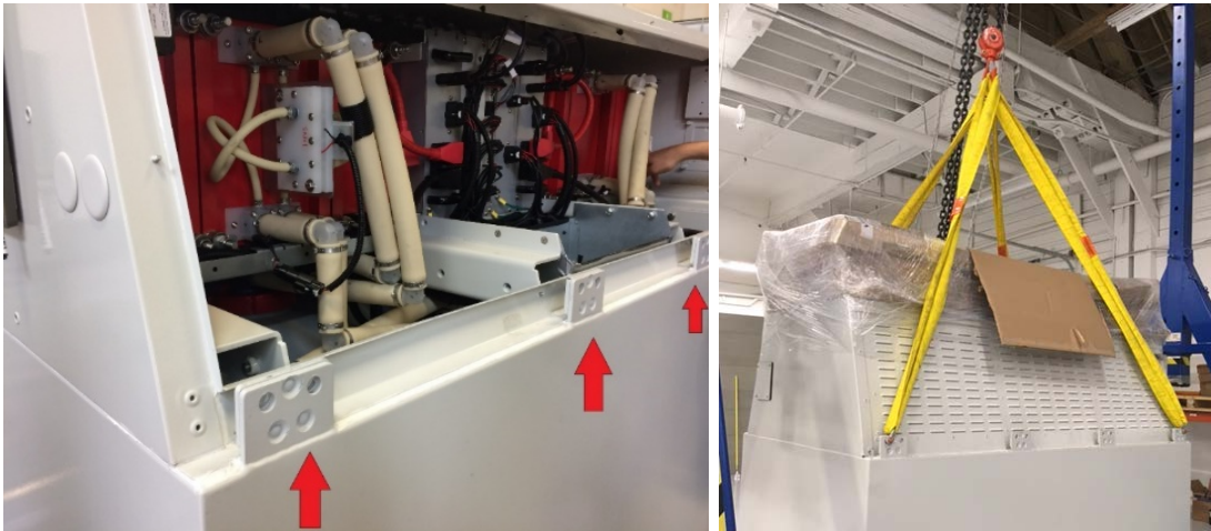
Figure 5 – Overhead lift points and example lifting arrangement.
