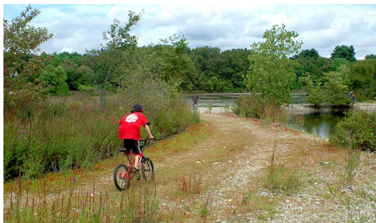
Figure 22: Gravel road approaching north end dike, 9/6/06
