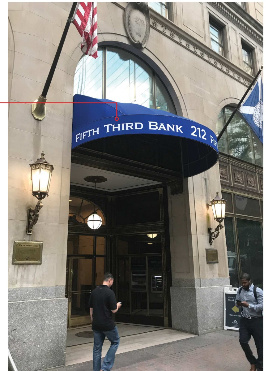
EXISTING BUILDING ENTRY CANOPY
