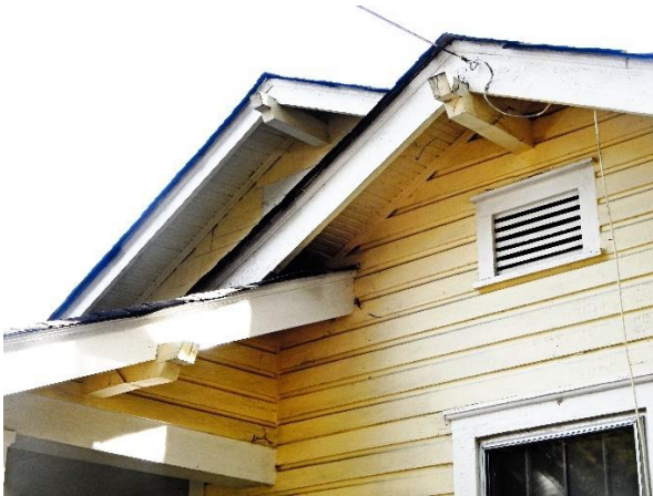
Exposed Tongue-and-Groove Roof Decking
