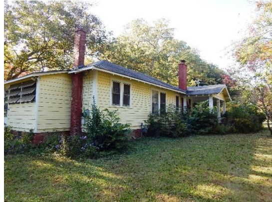
North Elevation Of House
