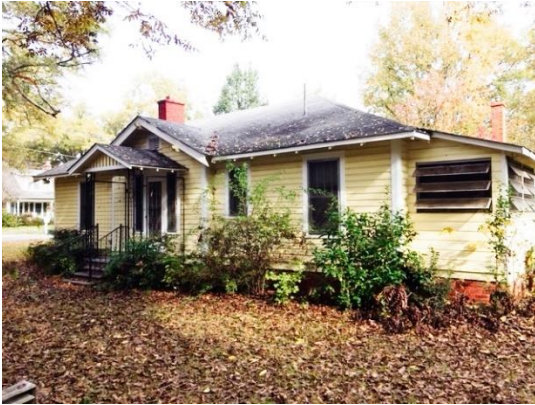
South Elevation Of House
