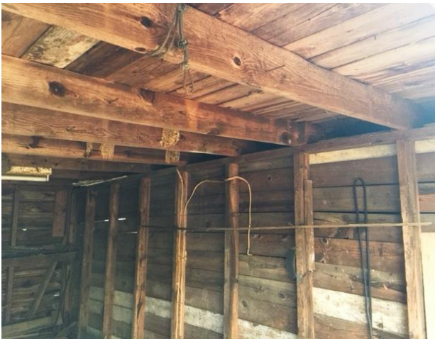
Exposed Inside Framing
