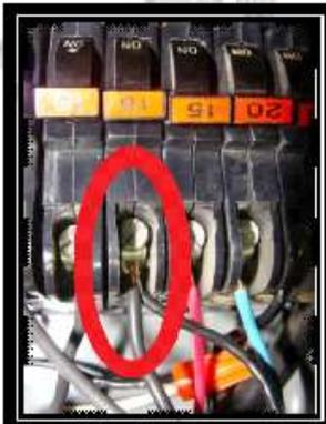
Furthermore, the wires could come loose at some point, one or both wires could have poor contact and/or circuit overloading can occur even if they feel very tight today. This can lead to over-heating, arcing, and possibly a fire.
