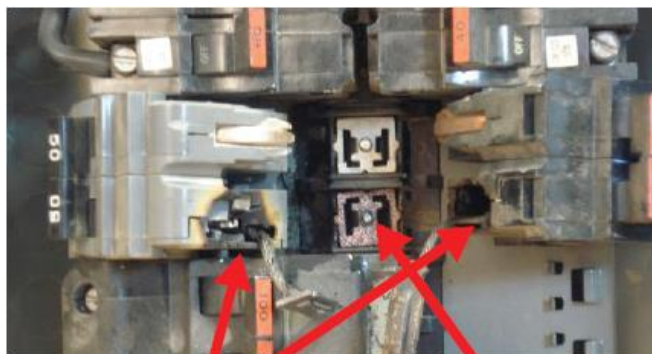
Burned breakers
