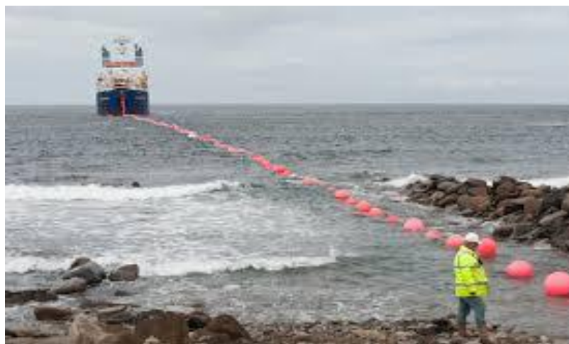
Figure 15 Cable laying at EMEC site, Ref.[1].
