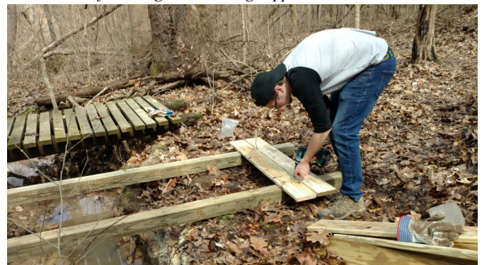
SIUC Geography student Jeremy Schultz replacing a footbridge with rotting supports at Fernlands Preserve
