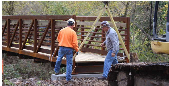
ET Simonds construction crew setting the 80' weathered steel pedestrian bridge
