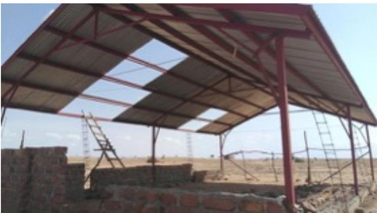
The church in Lodwar after the huge wind storm tore the roof off and knocked down the partially built walls.
