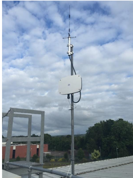
Figure 10 A LoRa gateway installed on the roof of the Cork pilot site.
