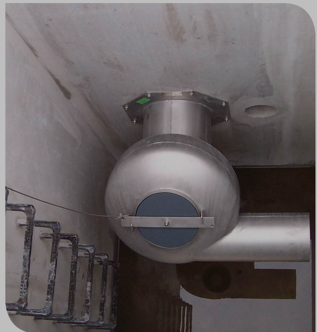
Figure 3: HYDROVEX® IHV EURO Typical Installation
