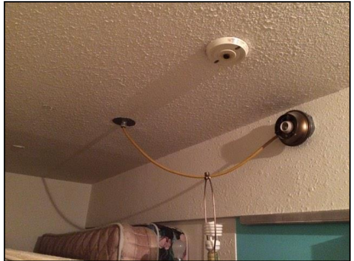
34. Exposed on walls or ceilings
