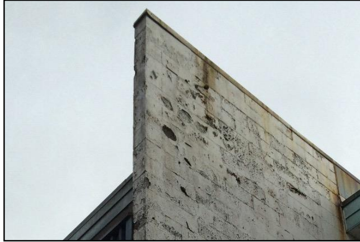
30. Masonry deterioration
