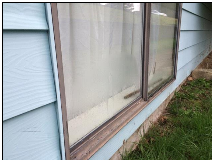
26. Excess condensation
