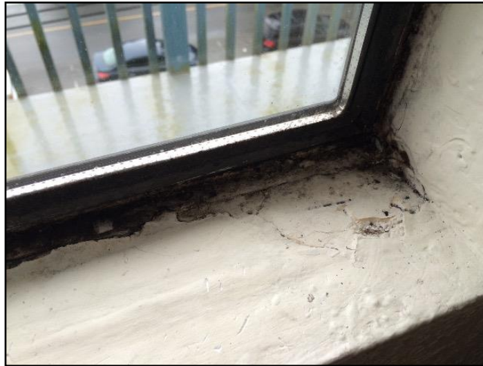
43. Excess condensation
