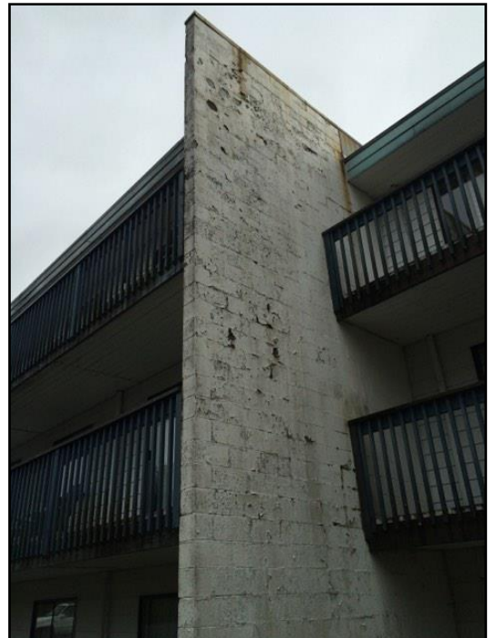
25. Masonry deterioration
