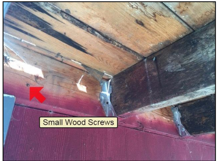
30. Screwed not bolted
