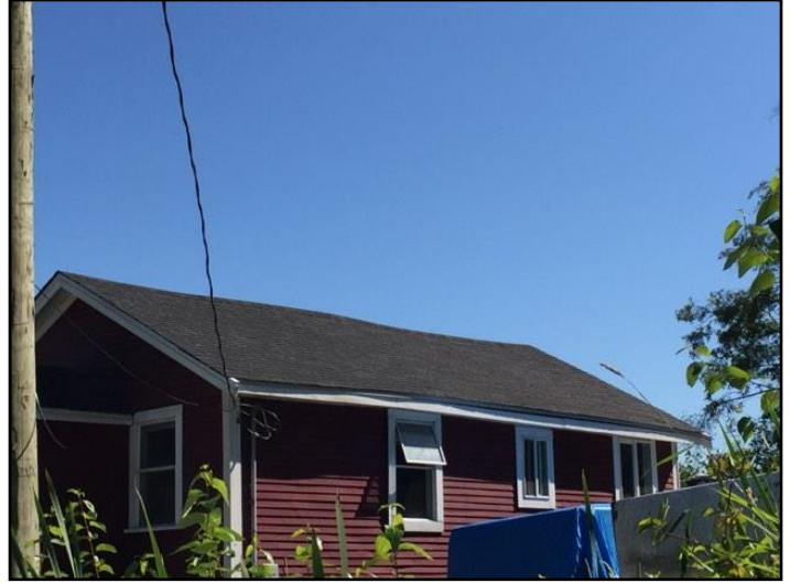
2. Asphalt shingles
