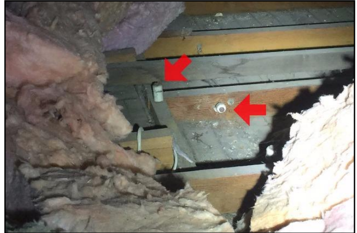
46. Copper - knob and tube
