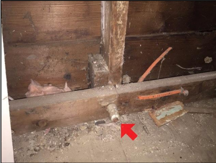
45. Copper - knob and tube
