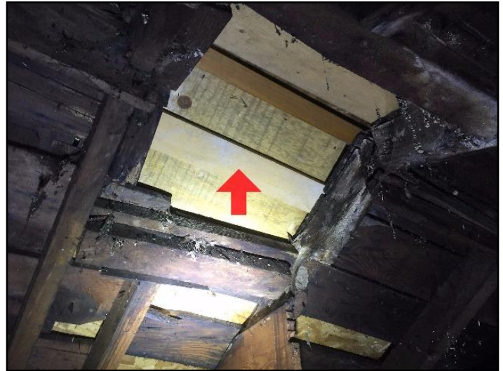
5. Patched where chimney used to come through
