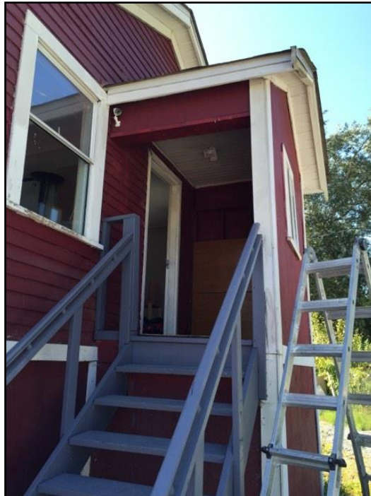
15. Wood Front Porch
