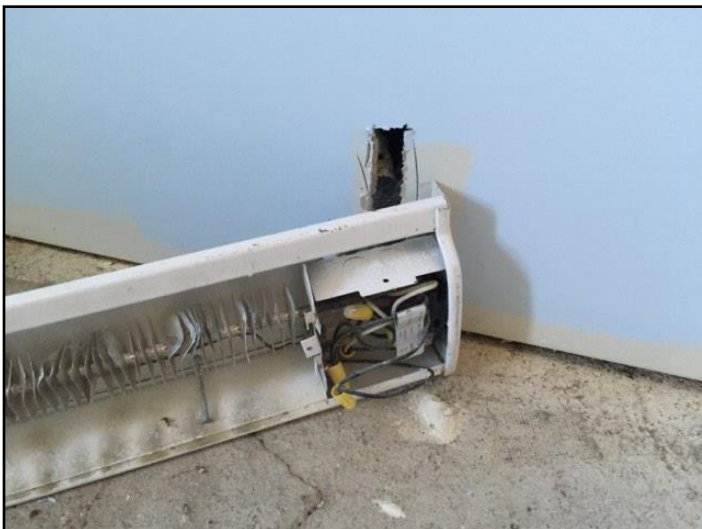
54. Exposed wiring
