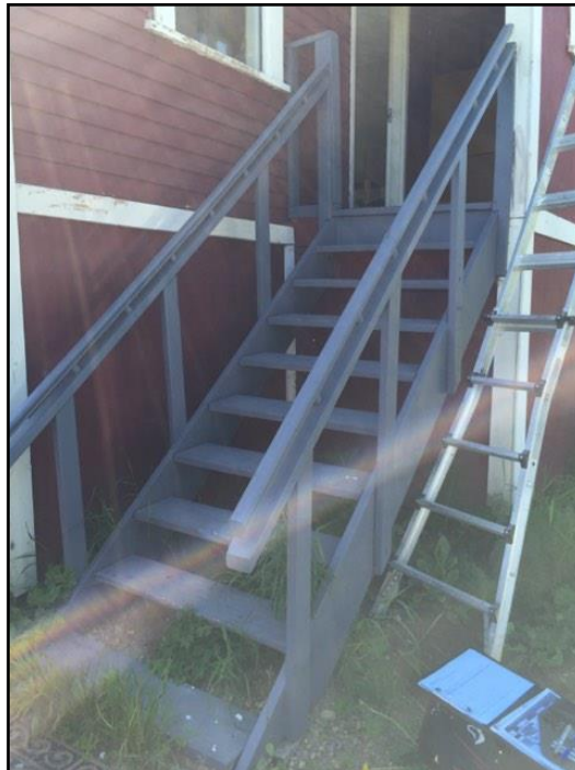
16. Wood Staircase - Front Door
