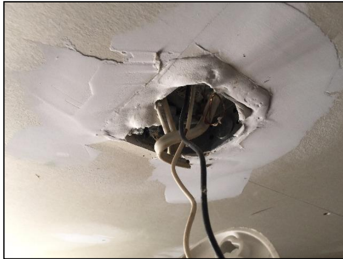
56. Exposed wiring
