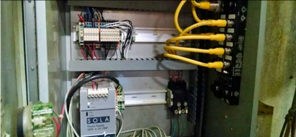
Figure 2: The field logic controller is at home in a control enclosure or out in a harsh environment.
